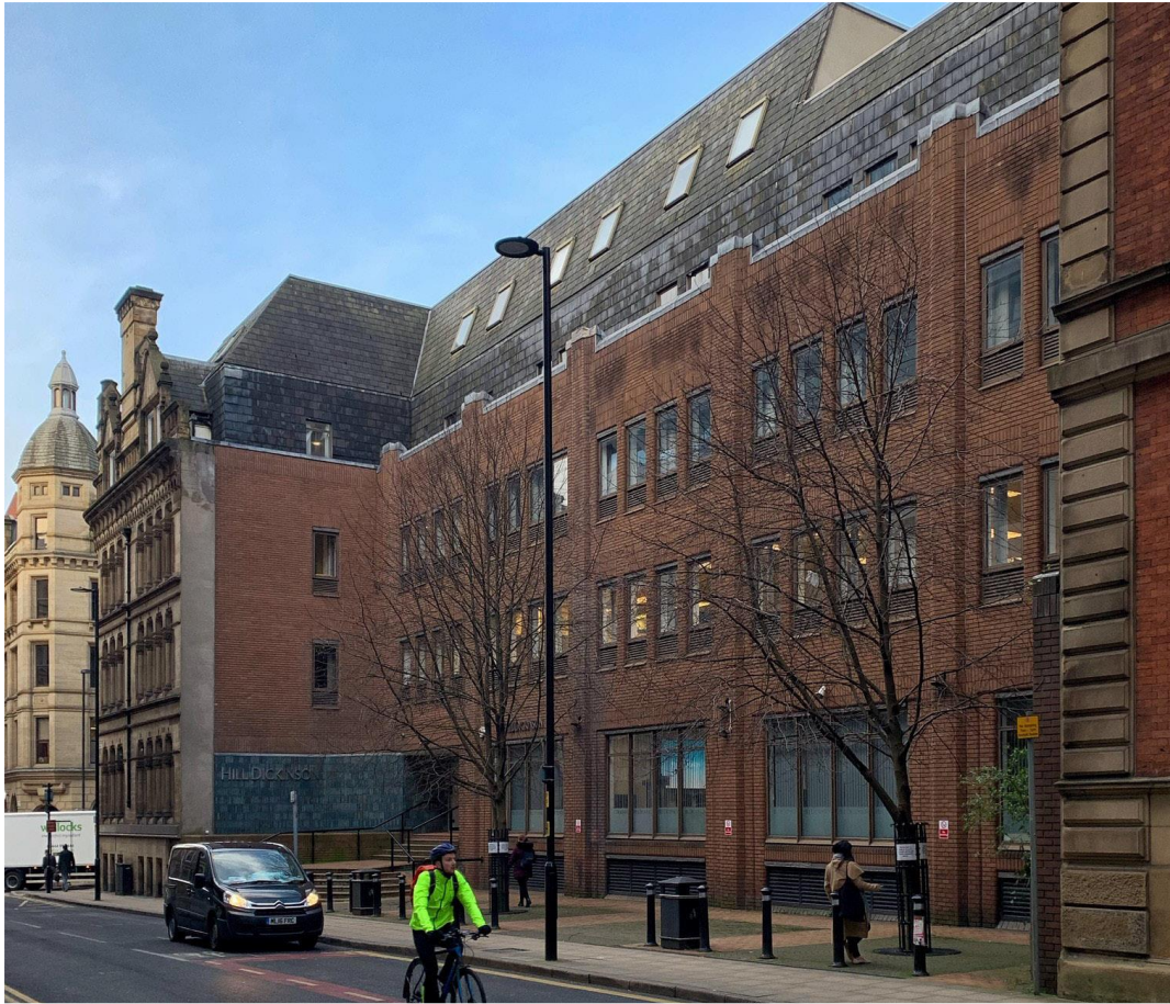
Figure 2 – View of Existing Building from Fountain Street
